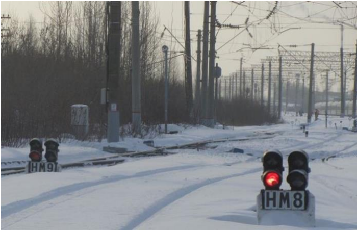
Part of Izhevsk station at winter time. You can see the switches cleaned but the tracks are not.
