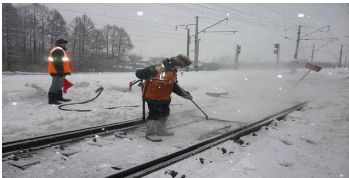
Cleaning the turnout by hose with compressed air
