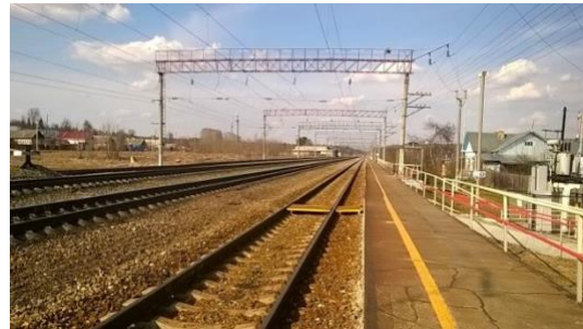
"The Usky station view to the north"
