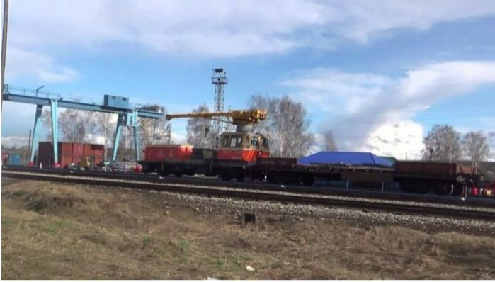
The maintenance diesel car with platform at the Pozim station
