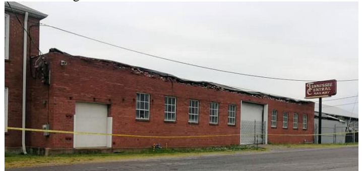
Photo by Jason Sharpe – Before demolition begins
