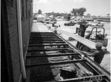
Digital photos above & below show the installation/rebuilding of the loading dock on the N side of our building. Jay "The Steel Man" Wilson & his lovely wife Michelle donated the \$1500 worth of steel to help make this possible. The 800 ft² dock frame was built of used rail and will be topped with a 4" deck of poured concrete. The work crew included Terry Bebout, Big Don Gage, Clarence Graham, Roy Poston, Gen Turnage & Jay Wilson. Digital Photos by Terry Bebout 1 July 2000.
